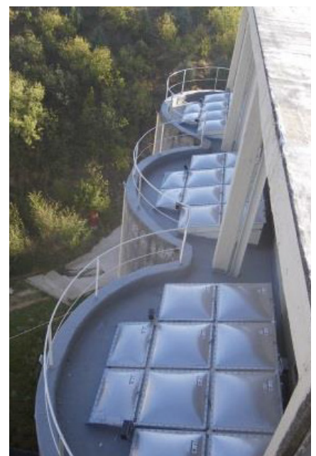
Vent panels on silo roof
